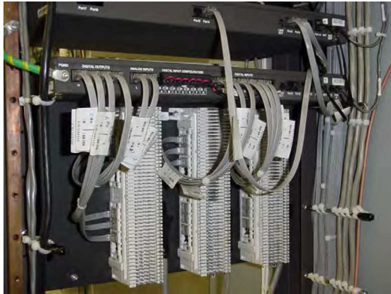
FIGURE 9-19 EXAMPLE OF CABLE LABELING
